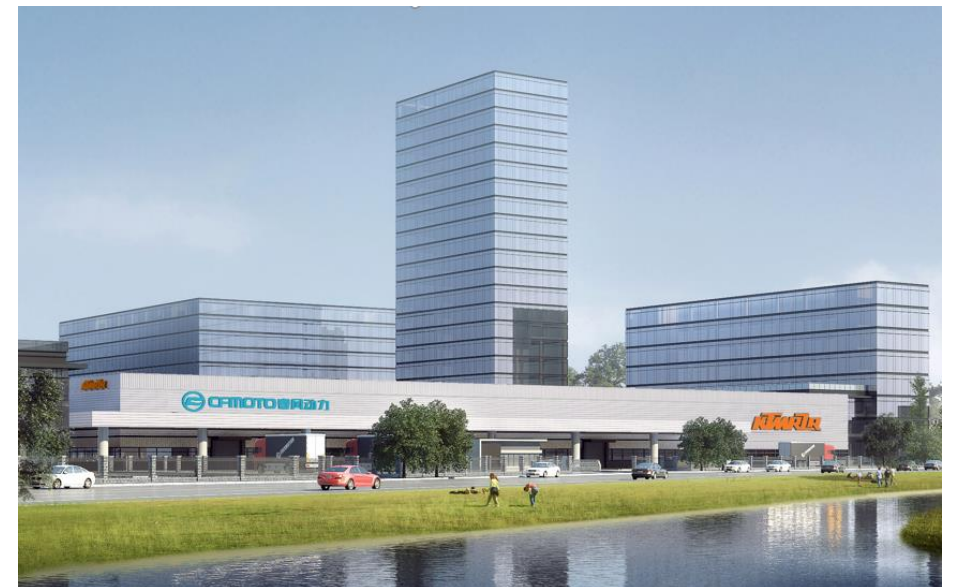
Plant under construction
